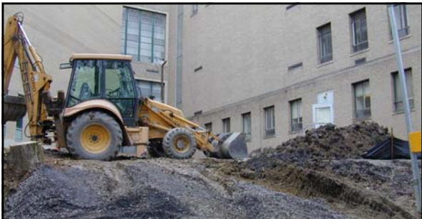
Sediment runoff rates from construction sites can be up to 20 times greater than agricultural sediment loss rates and 1,000 to 2,000 greater than those of forested lands.
